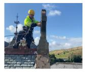
The stone cross above the front door is 'shaky' and will be taken down to be put back in place with secure non-ferrous fixings
