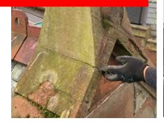
New lead flashings fitted to the wall of the next-door flats should stop water coming down into our big hall
